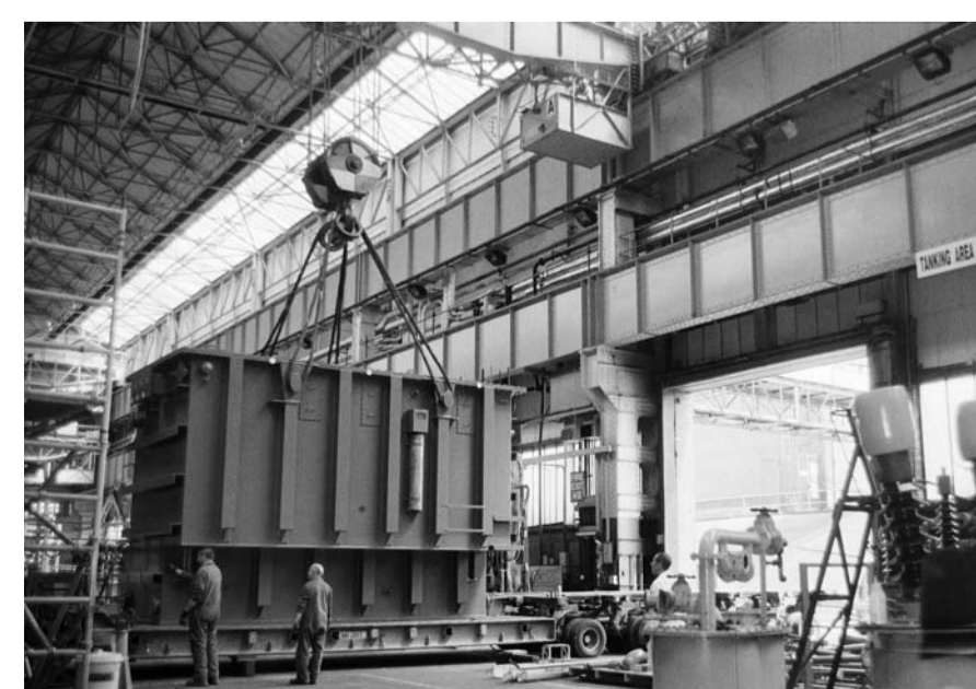
2003 Last transformer being loaded
